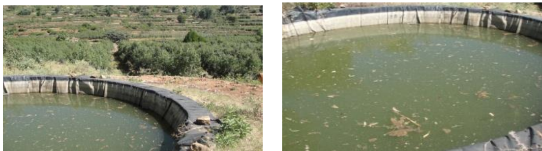
Figure 5: Sample of cylindrical rain-water-harvesting ponds pvc plastic
